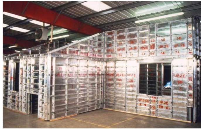
Fig1.Mivan Formwork
