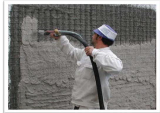
Fig 5.Shot creting over a wall
