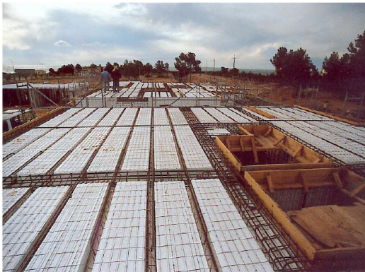
Fig 4.Placing of concrewall material.
